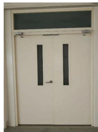
fire rated door with door closer, sequencer, small glass window
